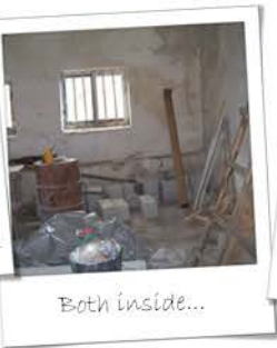
Lots of work to be done on the new shelter
